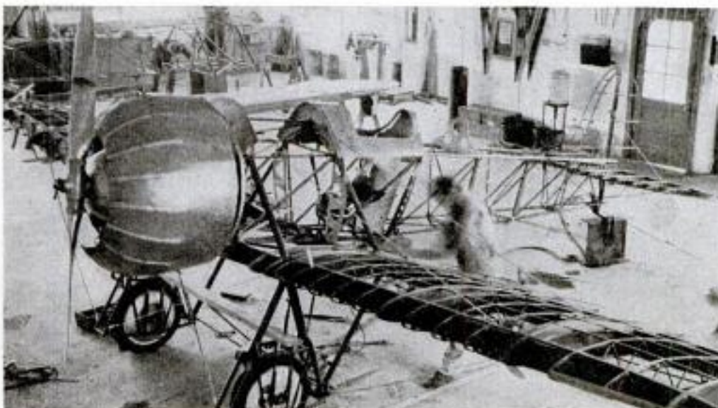
The "Mystery S" under construction, during which time all operations were carefully kept secret and withheld from the press.
